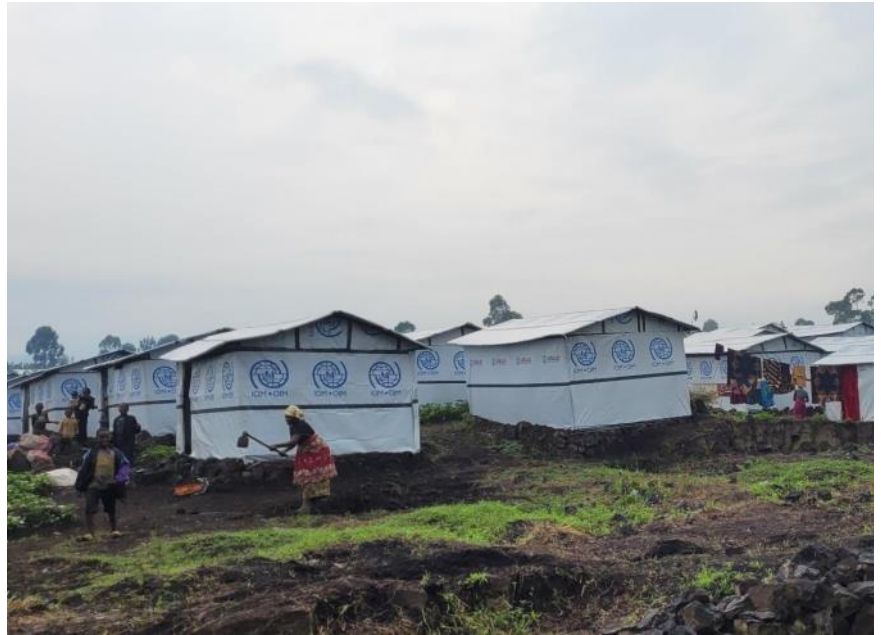
IOM constructed shelters in Rusayo II displacement site, Nyiragongo territory. / © IOM 2023
